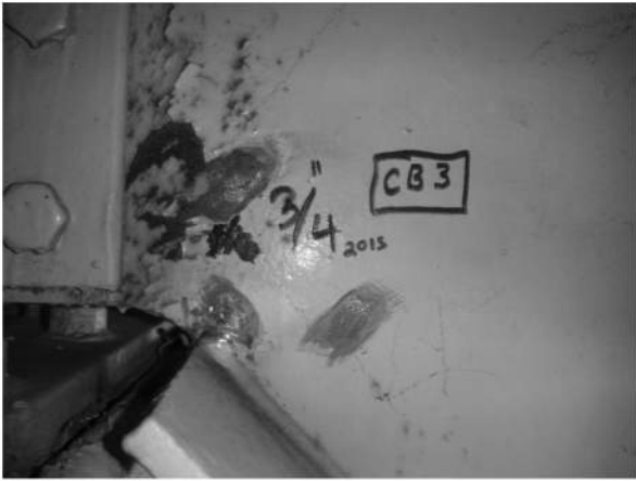
TYPICAL CB CRACK
