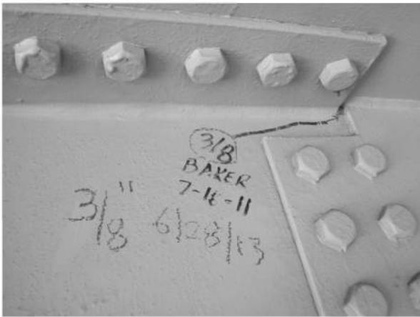
TYPICAL FT CRACK
