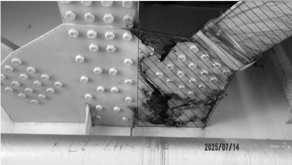
BOX GIRDER 74 – WEST FACE AT GIRDER E
