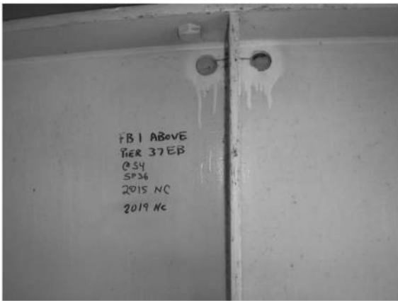
COMPLETED FS CRACK RETROFIT
