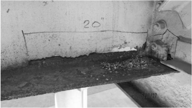
SECTION LOSS – GIRDER D
