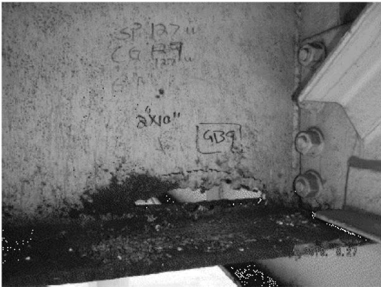
Photo 29 - Span 127W, Girder B, North face at cross-frame 1 - Hole through bottom of web (2" H x 10" L) - GB9
