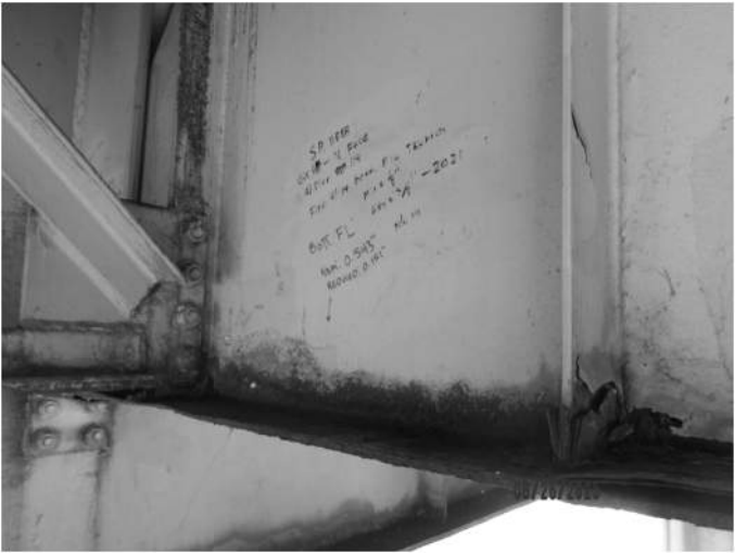
SECTION LOSS – GIRDER H
