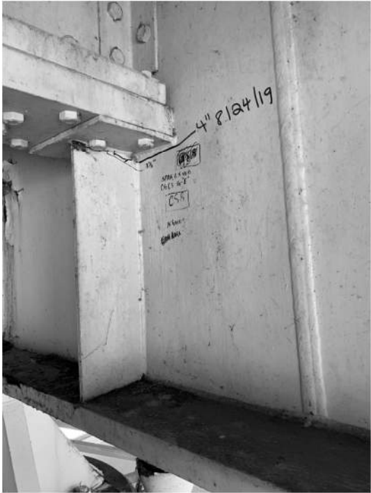
TYPICAL CS CRACK
