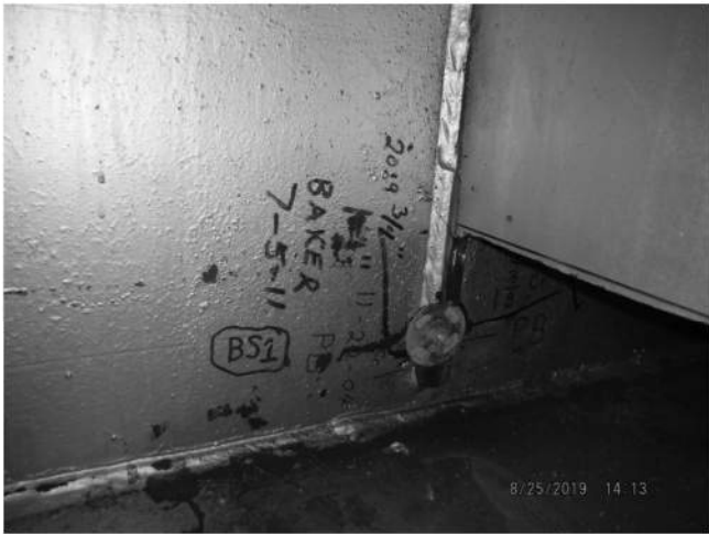
EXISTING BS1 CRACK RETROFIT
