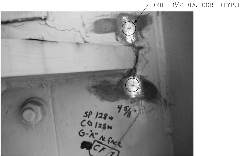
TYPICAL CF CRACK RETROFIT
