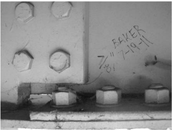
TYPICAL FB CRACK
