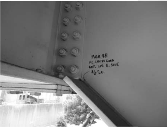
TYPICAL CB CRACK
