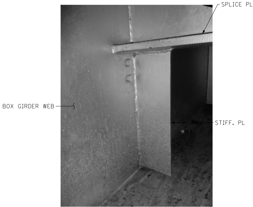
VIEW OF SPLICE PLATE AT PIER BOX GIRDER
