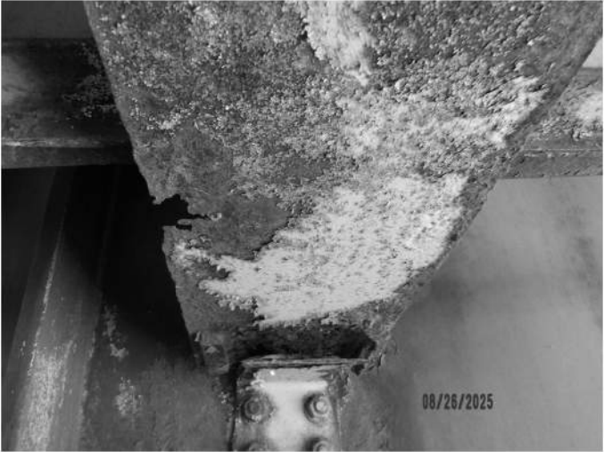
SECTION LOSS – GIRDER B BOTTOM FLANGE
