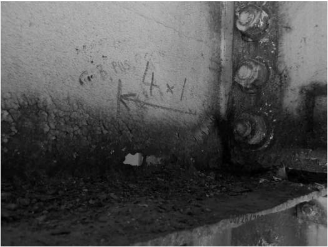
SECTION LOSS – GIRDER B WEB
