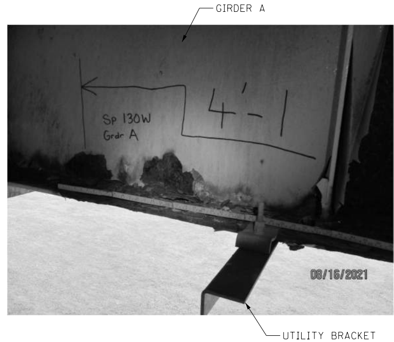
SECTION LOSS - GIRDER A
