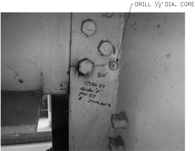
TYPICAL CC CRACK RETROFIT
